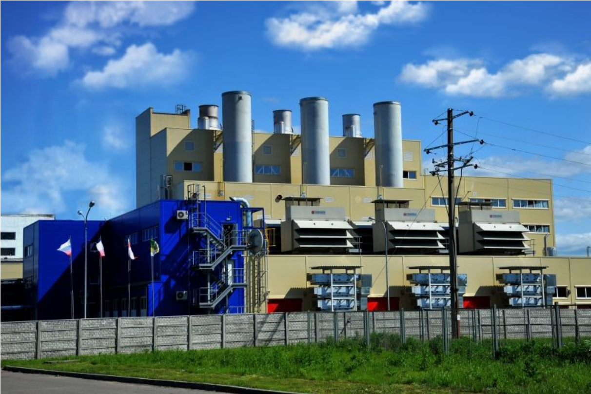
Figure 7. Combined cycle power plant - Krasavino 60 MW, Source: www.psg.eu
