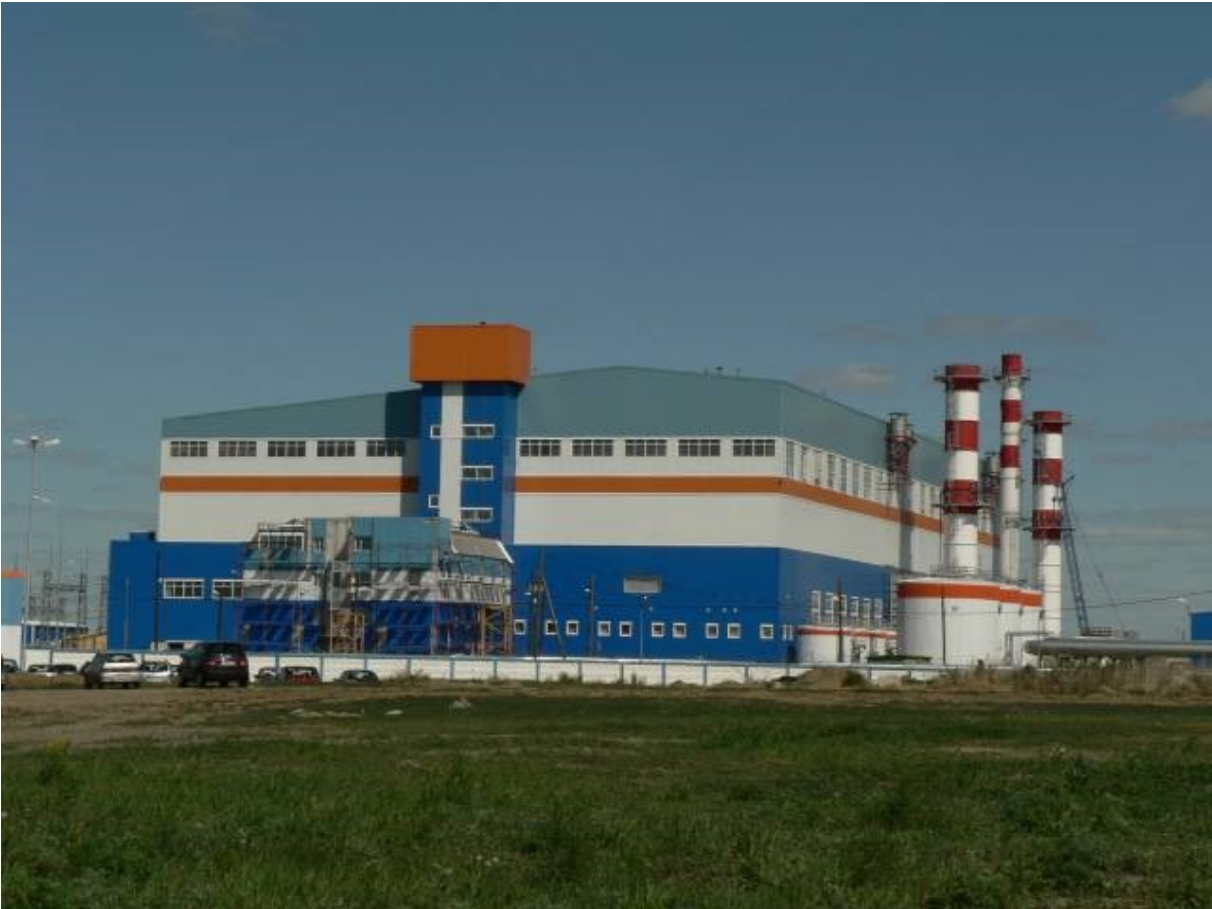
Figure 8. Combined cycle power plant – Kurganskaja TEC 229,5 MW, Source: www.psg.eu
